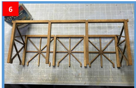
6 Glue the front frame on and leave to dry
